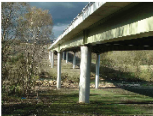
Bingley Bypass Viaduct spanning the River Aire
