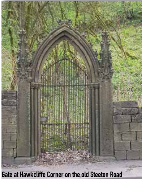
Gate at Hawkcliffe Corner on the old Steeton Road
